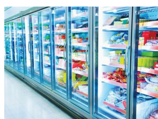
Refrigeration (-1 °C to 4 °C)
